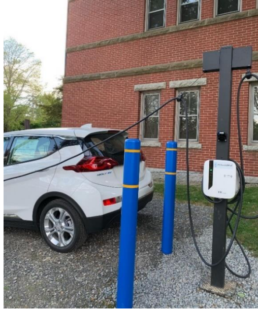
The Town of Kittery installed a two port Level 2 EV charging station at the Rice Library.
